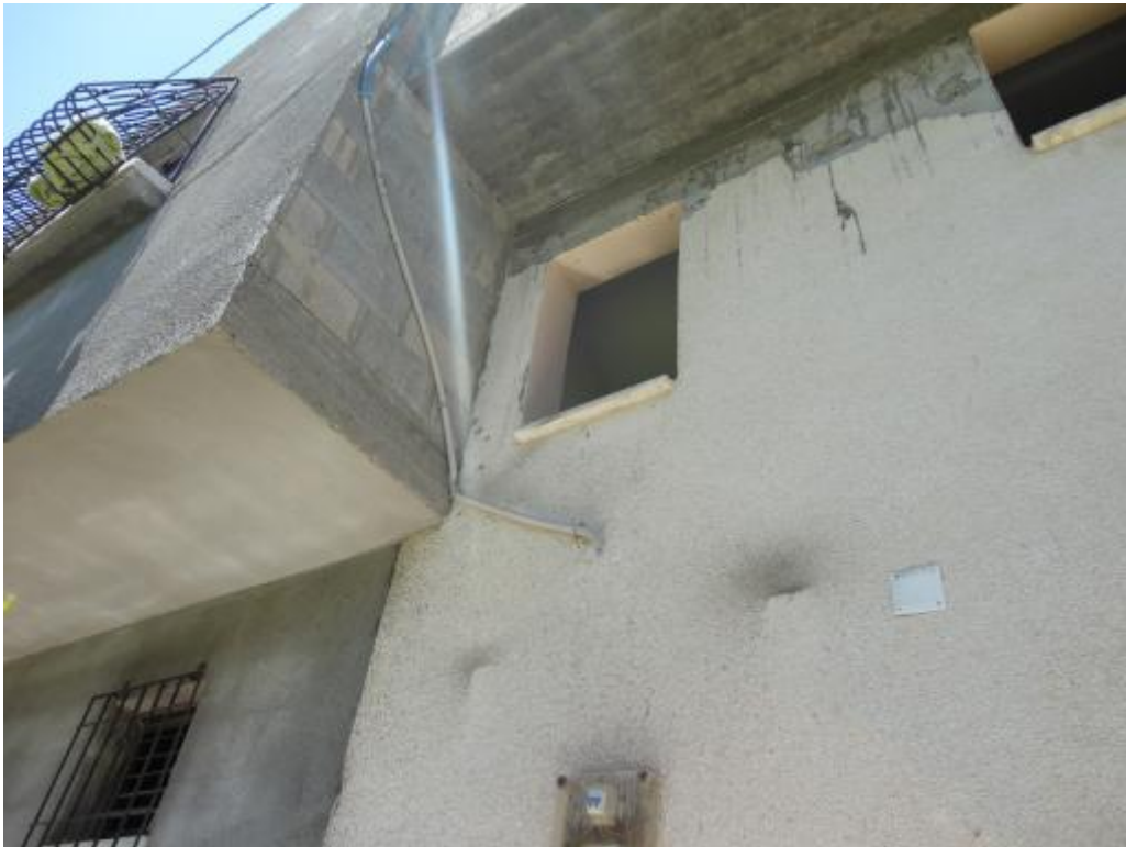
Changing the overall housing unit
