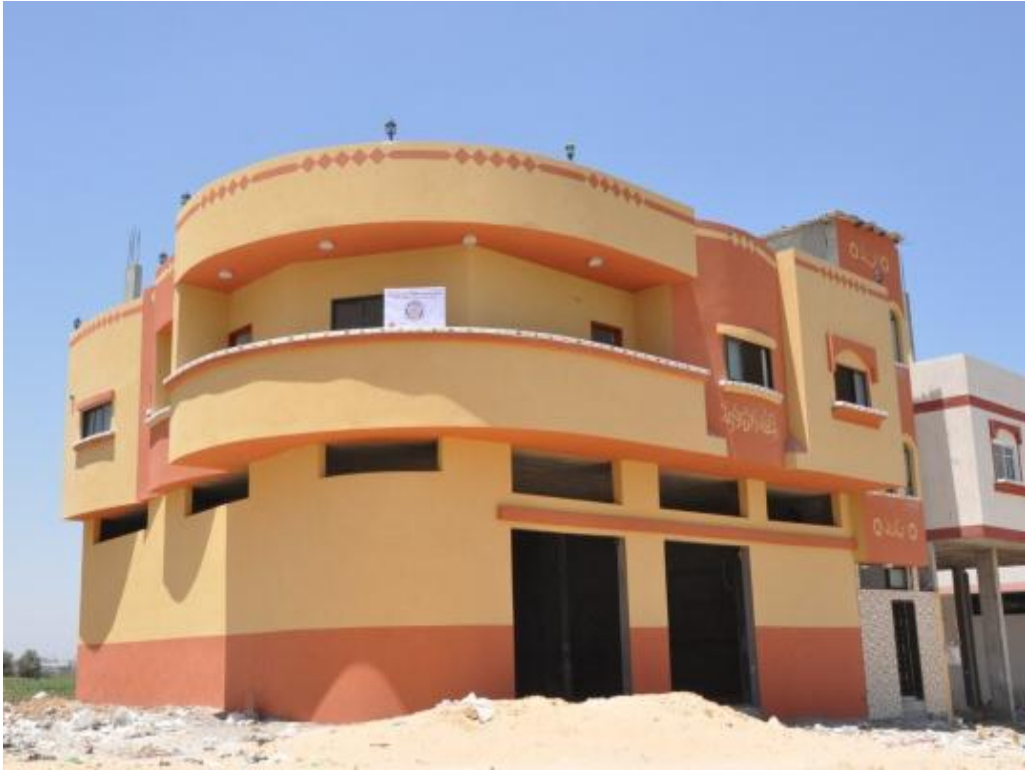
Completed housing unit Sammouni area / Gaza city - April 2013
