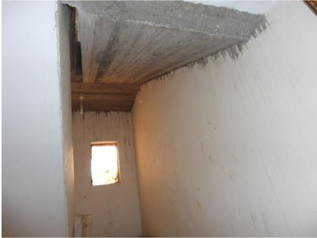
Adding stairs inside the housing unit Sammouni area / Gaza city - April 2013
